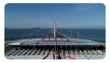
Hongkong-Zhuhai-Macau bridge construction commenced since 12/2009 and completed in 09/2018,totaling 55KM long with bridge and marine tunnels. 4man-made islands are composed by thousands of marine piles.
